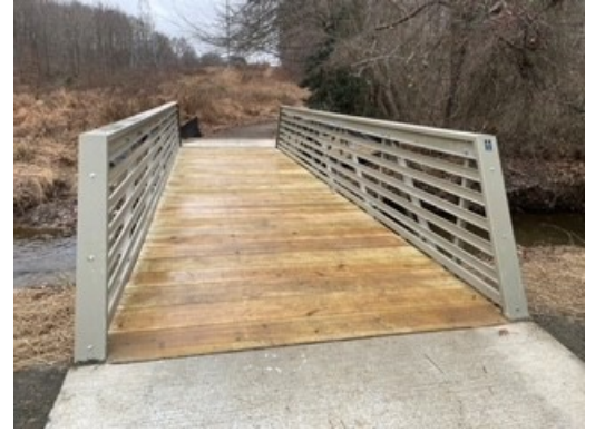
Photo of sample bridge
