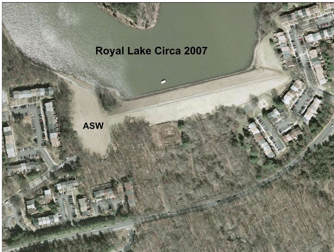
Figure 5. Royal Lake Dam and Spillway Circa 2007
